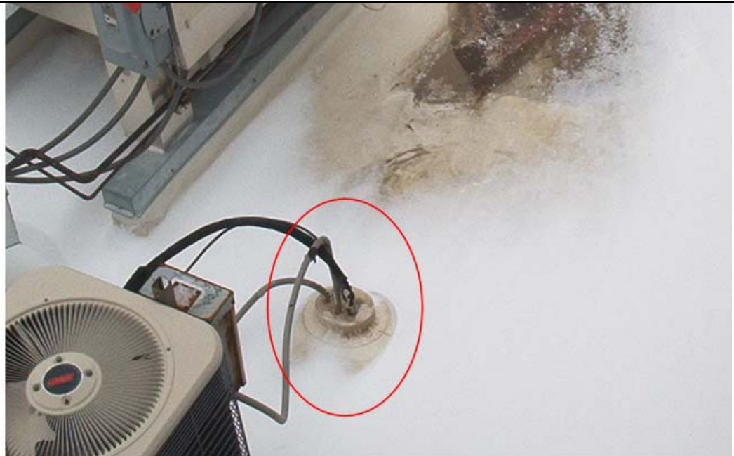
Site A rooftop penetration location
