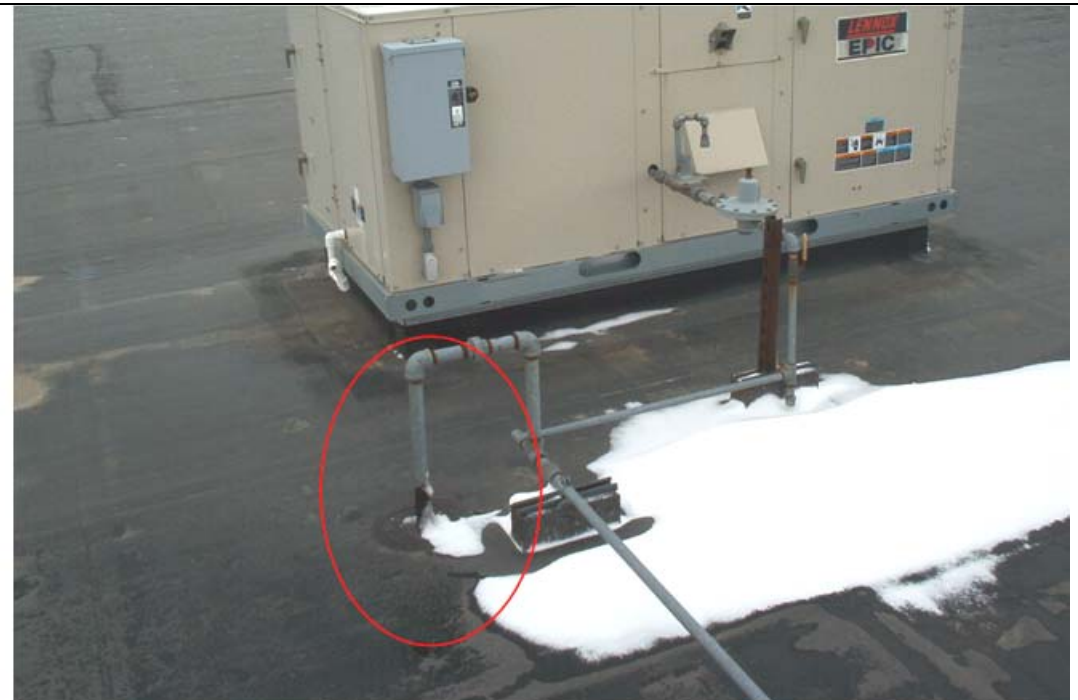
Site B rooftop penetration location
