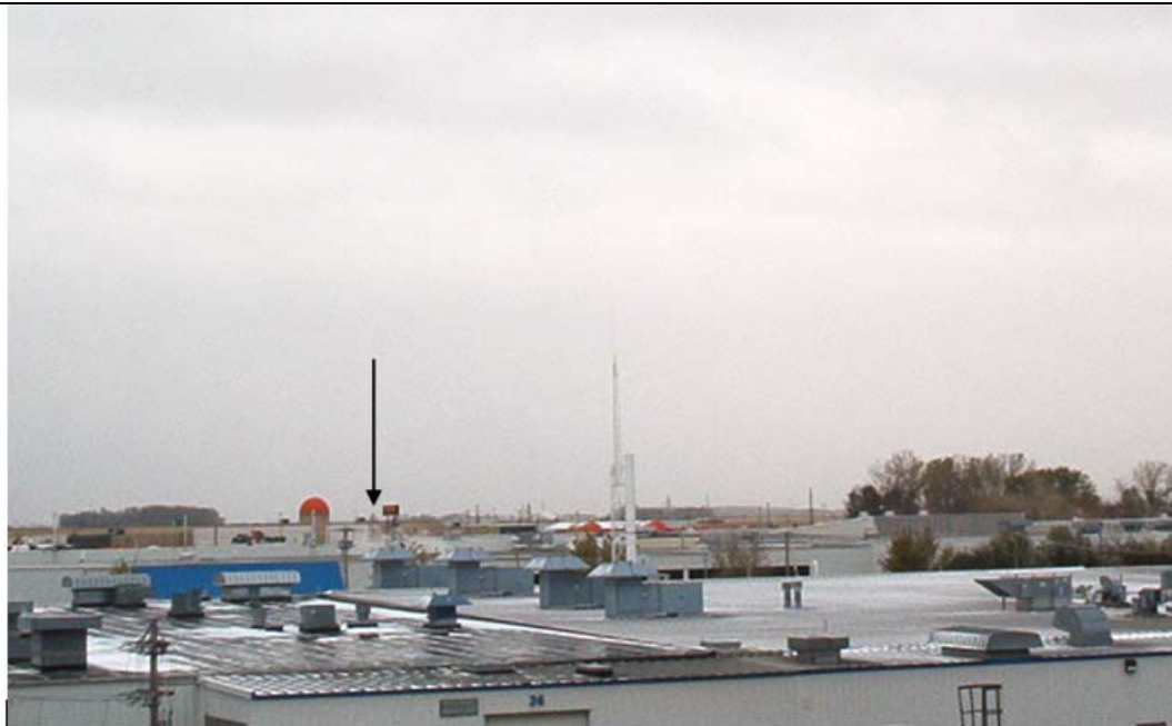
Site A rooftop line-of-site view looking at Site B
